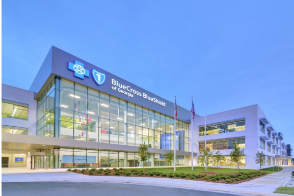
Blue Cross Blue Shield Columbus, GA Size: 243,000 SF Three-story office building
