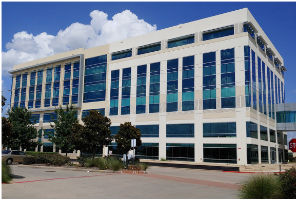
Katy Ranch Crossing Katy, TX Size: 2 buildings each 156,000 SF Six-story stacked tilt panel office building and garage
