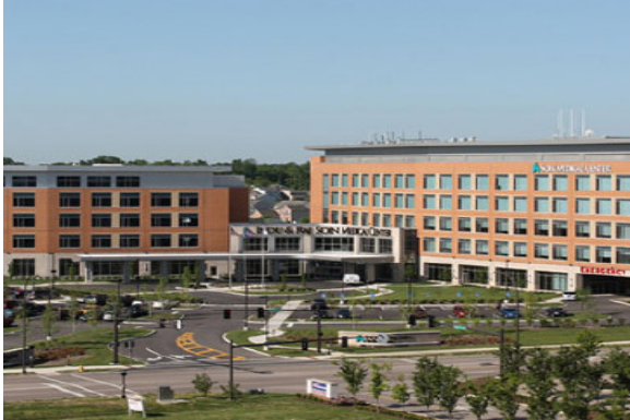
Ollie Davis Medical Pavilion Beavercreek, OH Size: 100,000 SF Five-story medical office connecting to adjacent hospital
