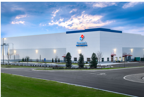
Domino's Supply Center Lexington, SC Size: 67,200 SF Distribution center with three coolers
