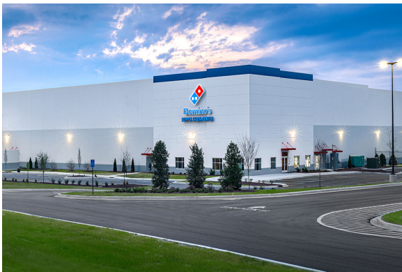
Dominos Supply Chain Center Lexington County, SC Size: 67,800 SF Distribution center with three coolers
