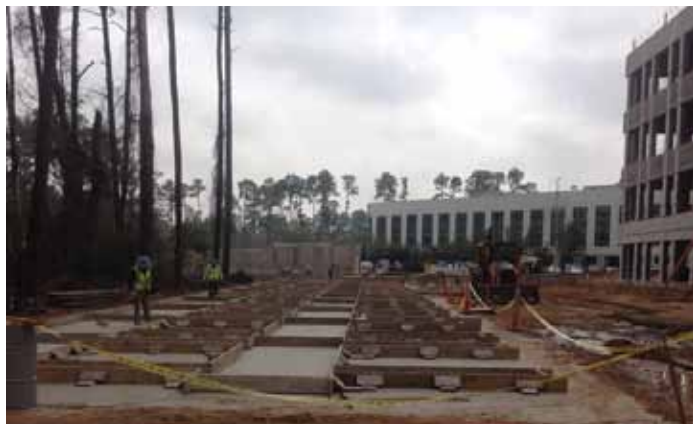
Phase 2 east side framed panels. Courtesy of E.E. Reed Construction, L.P.
